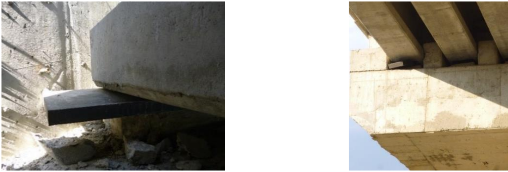
Figure 19. Displacement of elastomer bearings
