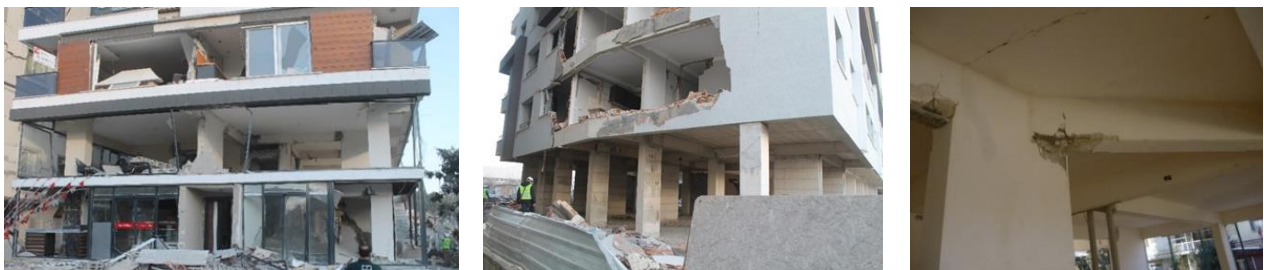
Figure 2. Discontinuities in the axis system
