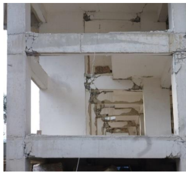
Figure 4. Slab discontinuities
