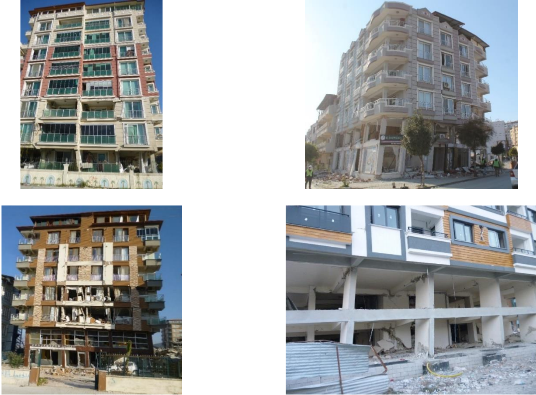
Figure 3. Weak/soft story mechanisms
