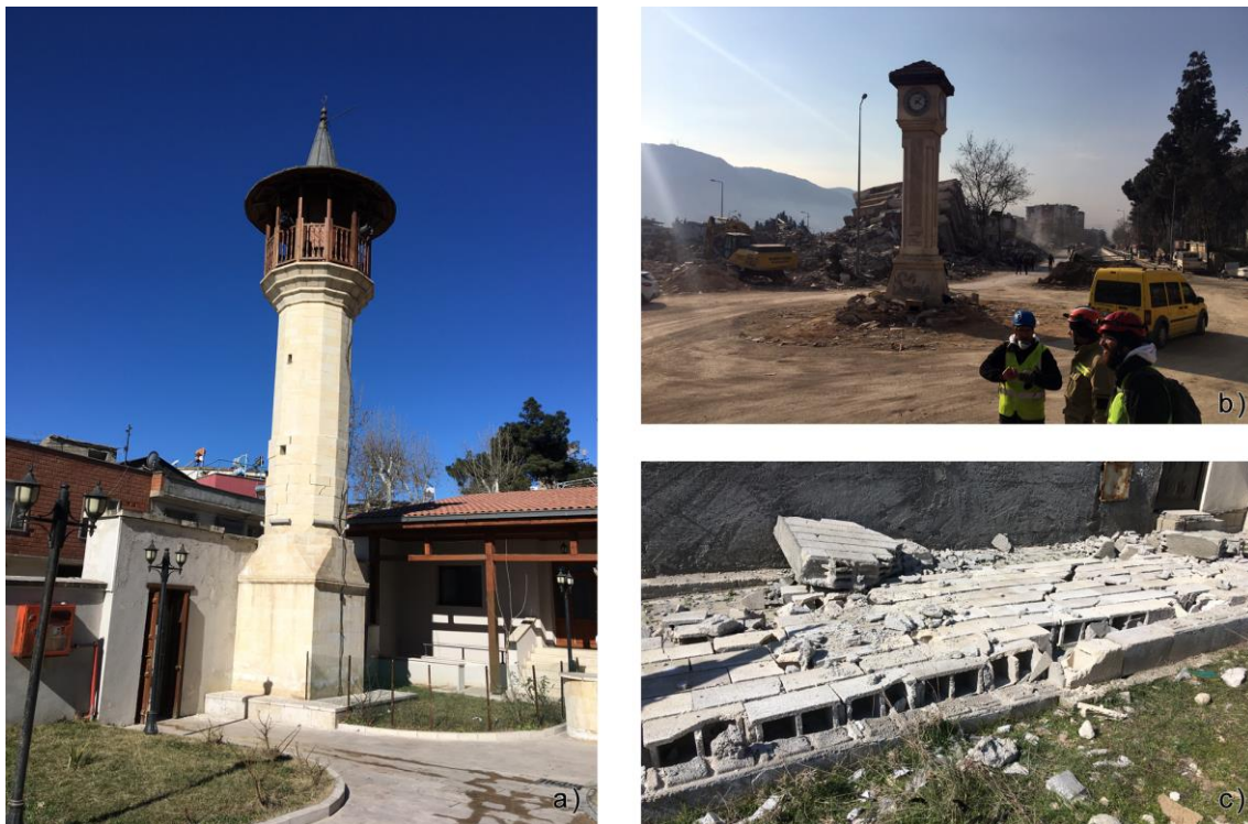
Figure 3. Damaged or ruined rocking structures in Kahramanmaraş (a, c) and in Antakya (b)
