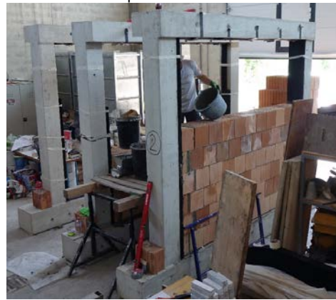
Step 3: Brick laying
