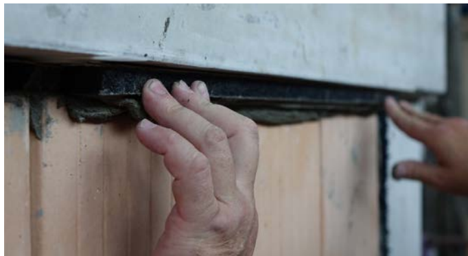
Step 4 – Insertion of outer rubber stripes at the top
