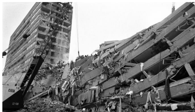
Figure 2.2 Building collapse during the September 1985 earthquake. (PEINADO, 2012)
