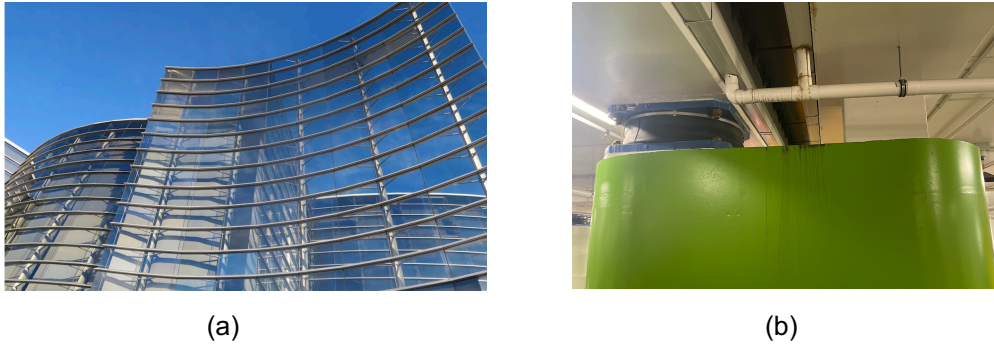
Figure 3. Christchurch Art Gallery: (a) Global view; (b) Base isolator in the underground
