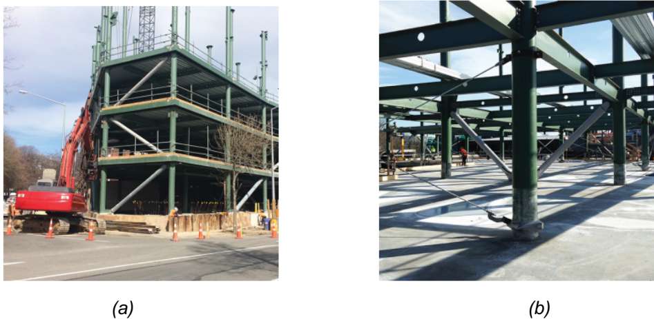
Figure 6. PwC Centre: (a) Architecture view (Courtesy of Beca); (b) Close-up view of bracing (Courtesy of Steel Construction New Zealand)
