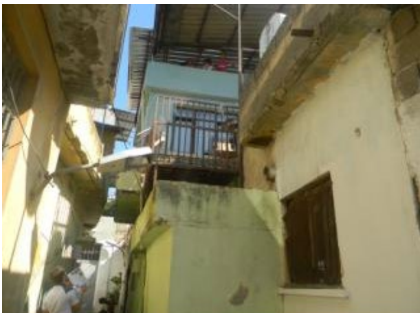
c) Masonry buildings with irregularities in elevation
