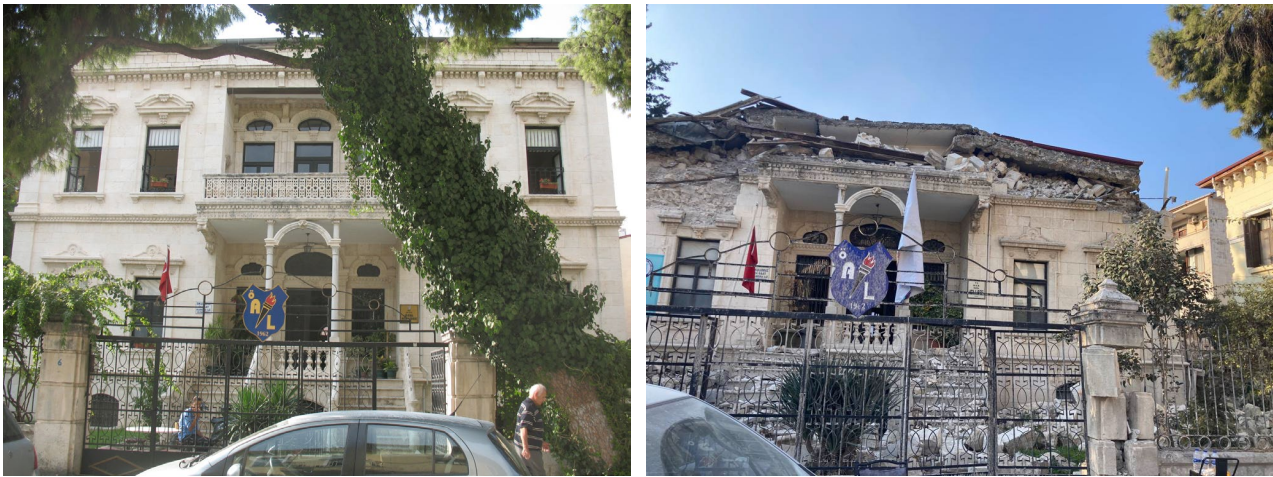
a) Masonry school building before and after the earthquake
