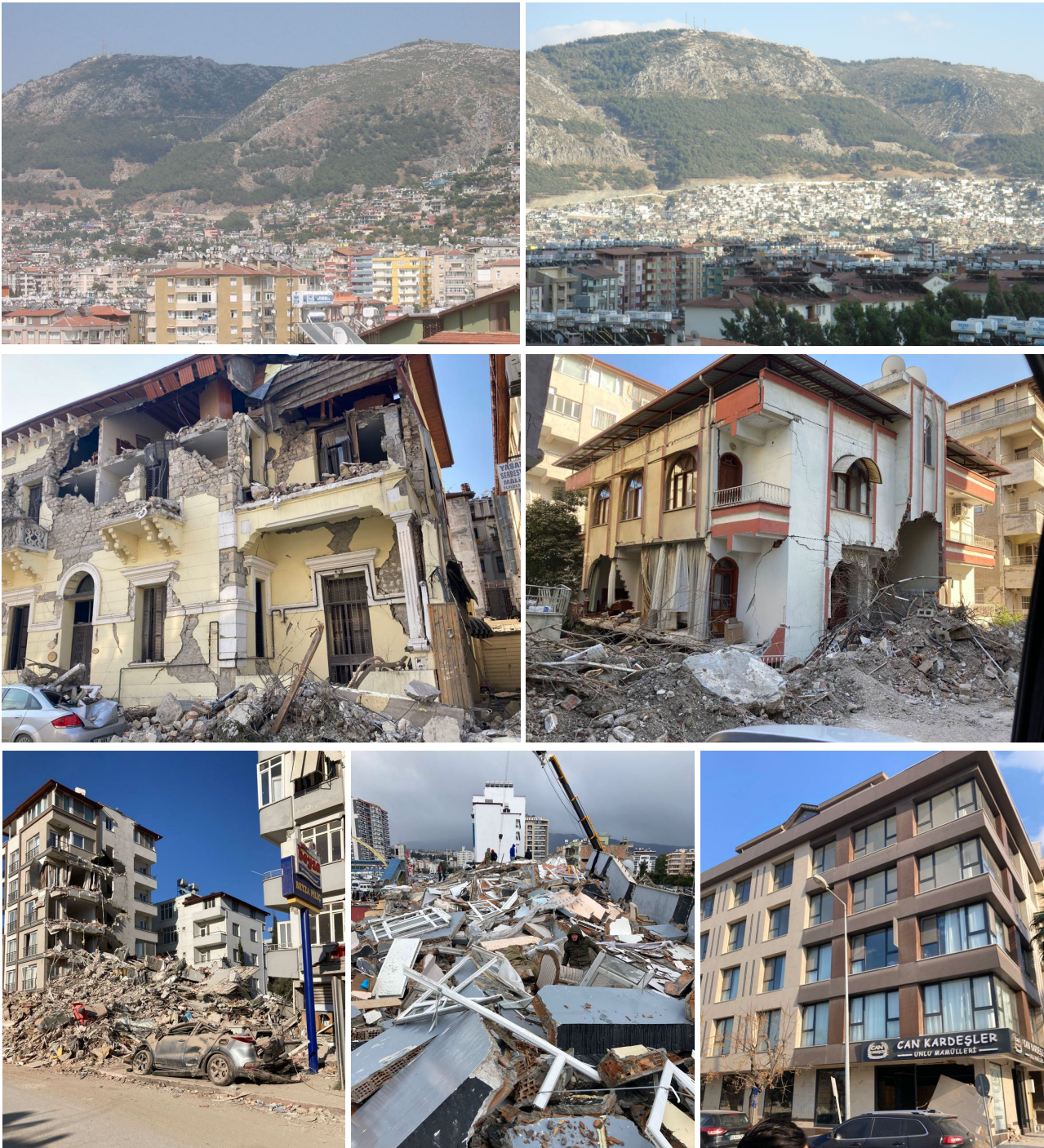
Figure 1. Sample pictures of Antakya's building stock and recent damages (© EDAC & M.C. Genes).
