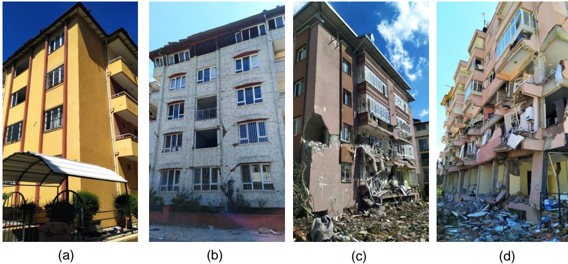
Figure 6. Examples of mid-rise Reinforced Concrete (RC) building damage observations from all damage states: (a) DS1 S and DS1 NS , (b) DS2 S and DS2 NS , (c) DS3 S and DS3 NS , (d) DS4 S and DS4 NS .
